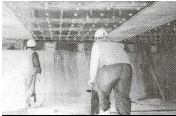
Figure 5.59: Epoxy injection in building retrofit
