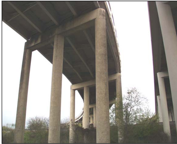
Figure 4.3: Southern Pacific Railroad and FM 78 bridge, showing typical high clearance
