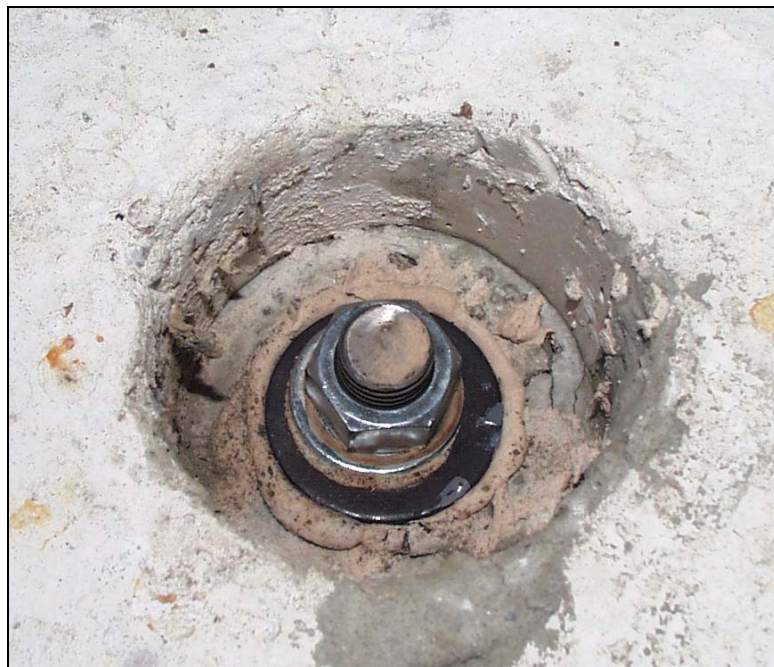
Figure 5.33: Welded Threaded Rod with HY 150 adhesive beneath the washer
