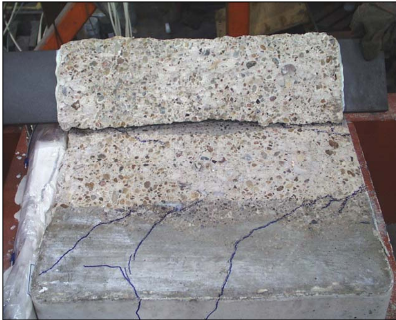
Figure 6.5: Epoxy Plate failure of the concrete below the adhered surface
