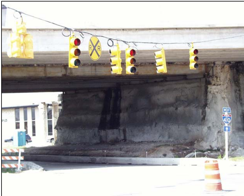
Figure 4.16: Honeysuckle Lane bridge during demolition
