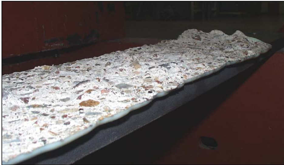
Figure 8.15: Concrete remaining adhered to steel plate after failure
