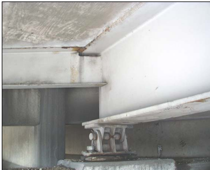
Figure 4.6: Roller-rocker support at abutment of Huebner Road bridge
